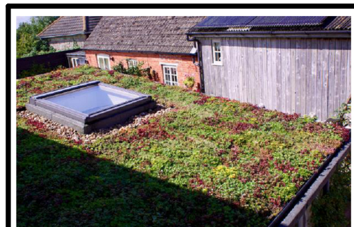
Sedum and Moss Roof to Enhance Biodiversity
